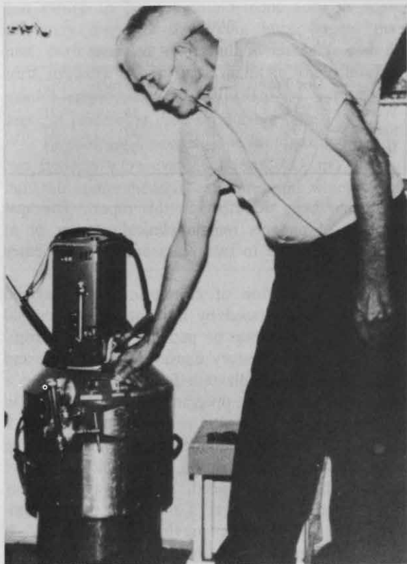
Fig. 4—Linde oxygen walker system. Lower container has approximately 3½ days oxygen supply. This can be used directly or used to fill the 7.5 pound canister which the patient uses for ambulatory oxygen therapy.
